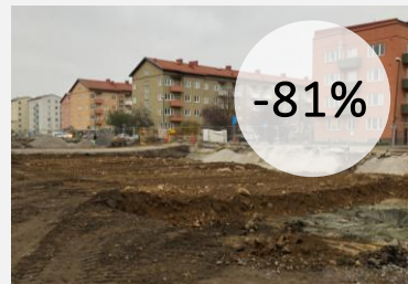
Jernhusen Marksanering, Malmö
