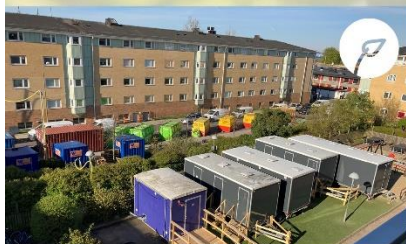
Kv. Piggvaren 10, Limhamn Stambyte & badrumsrenovering: 97 lgh
